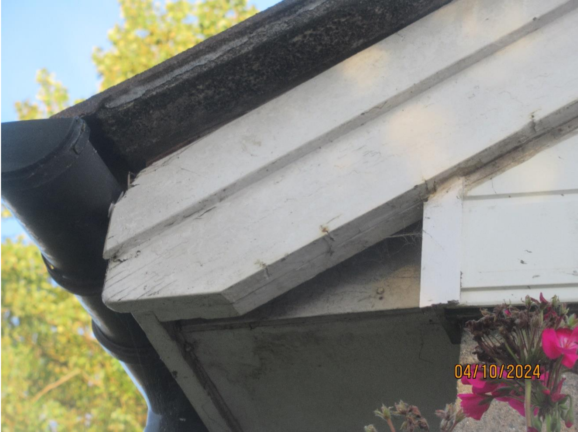
P12 – depot soffit
