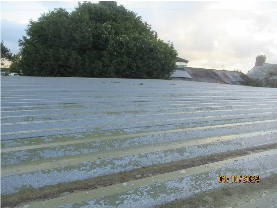
P6 – Maurice Huggins roof
